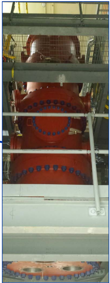
PFBC Pressure Vessel
